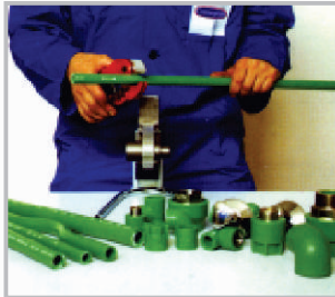
Cut required length with cutter
