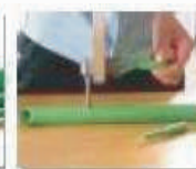
(Repair process of hole repair bar)
